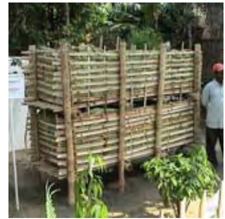
Bladder tank 3000 liter in bamboo construction: 0.6 Taka per liter construction cost, and incl. supply chain profit WHO, 2002
