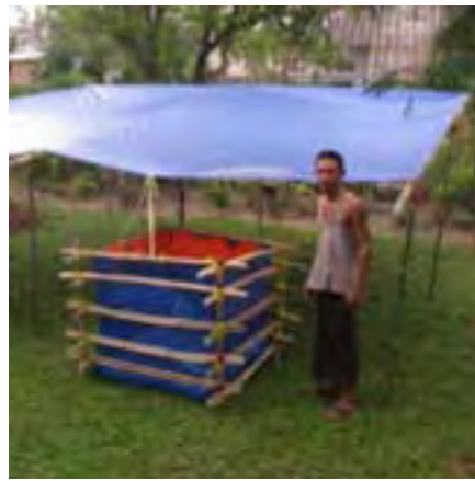
IDE-Myanmar's tarpaulin system uses bamboo framing to support their storage bag and runoff frame.
